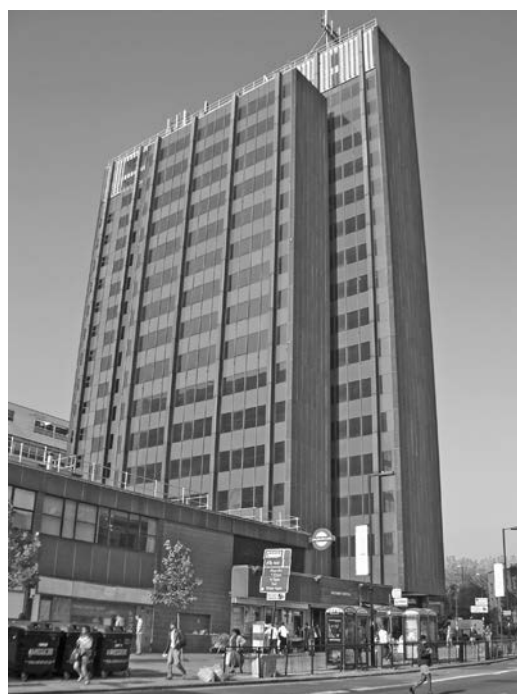
Archway Tower and Tube station, London.
